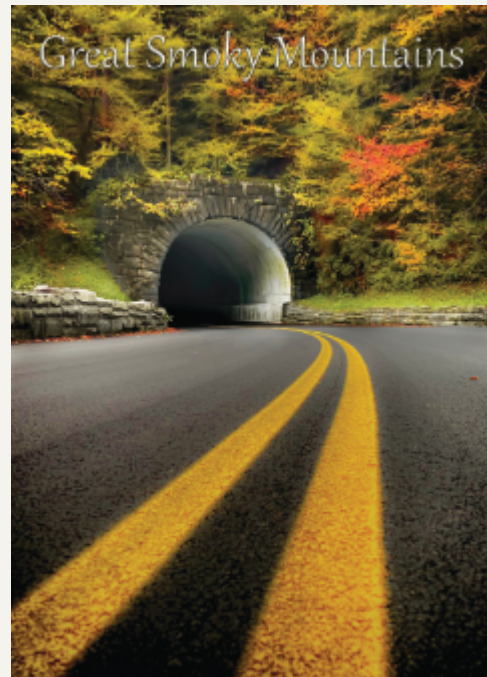
Fall Through the Tunnel
